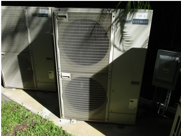
The 4 Ton Mitsubishi Condenser Unit 2 (CU 2) is at the North exterior Wall. It was manufactured in 2014 and was installed in 2015. It is paired with the two Air Handlers below.
