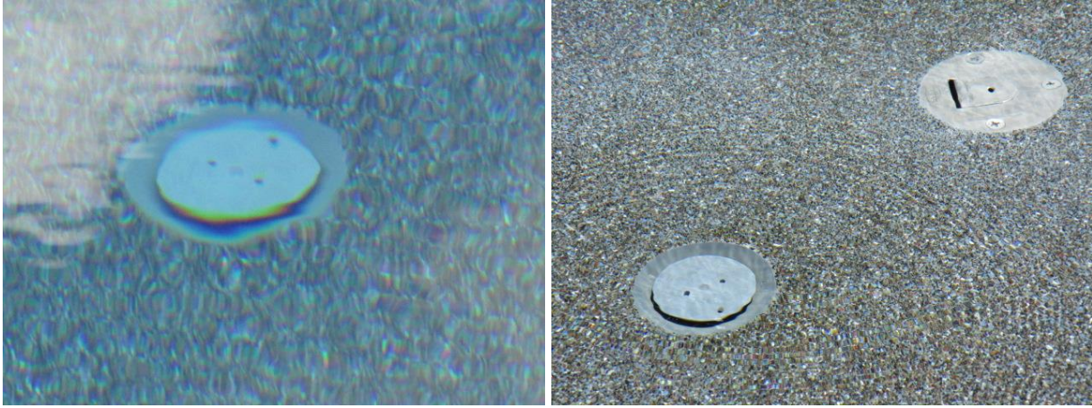
The Drain Covers were in good condition
