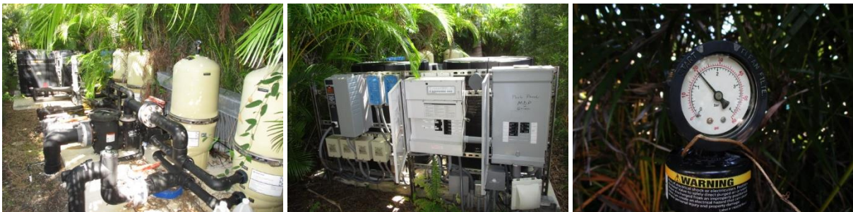
The Pool Pumps, Filters and Control Panels appeared functional
