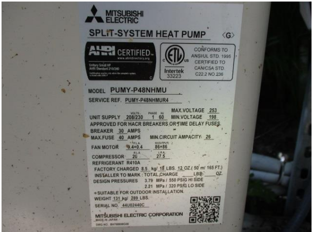
The 4 Ton Mitsubishi Condenser Unit 2 (CU 2) is at the North exterior Wall. It was manufactured in 2014 and was installed in 2015. It is paired with the two Air Handlers below.
