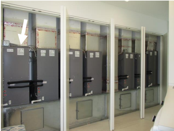
Air Handler Unit 3B (AHU 3B): Mitsubishi | 1.5 Ton | 2011 (installed in 2015) | The Air Handler is in the second-floor Utility Room
