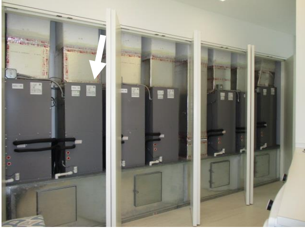
Air Handler Unit 3A (AHU 3A): Mitsubishi | 1 Ton | 2010 (installed in 2015) | The Air Handler is in the second-floor Utility Room
