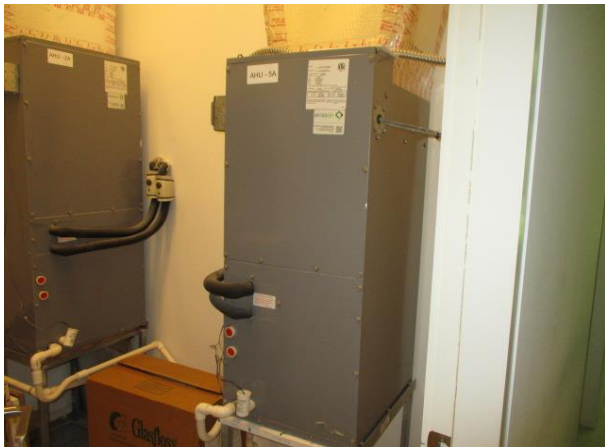
Air Handler Unit 5A (AHU 5A): Mitsubishi | 2 Ton | 2011 (installed in 2015) | The Air Handler is in the first-floor HVAC Room
