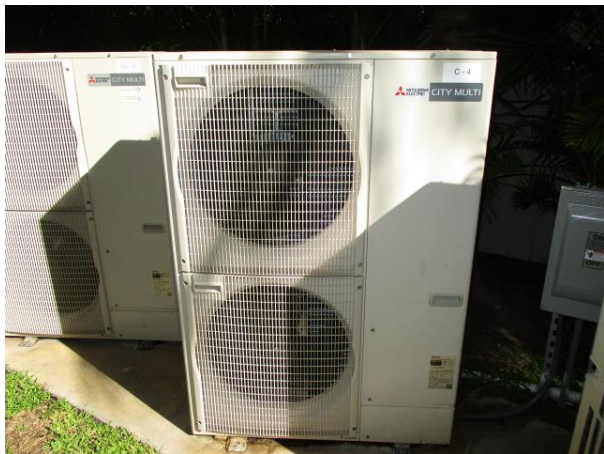
The 4 Ton Mitsubishi Condenser Unit 4 (C 4) is at the North exterior Wall. It was manufactured in 2014 and was installed in 2015. It is paired with the two Air Handlers below.
