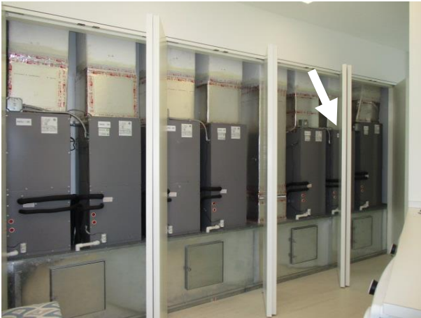
Air Handler Unit 1A (AHU 1A): Mitsubishi | 1.5 Ton | 2011 (installed in 2015) | The Air Handler is in the second-floor Utility Room
