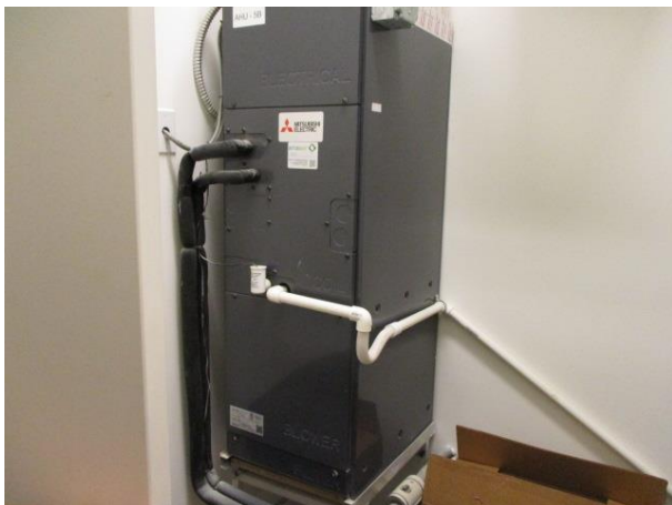
Air Handler Unit 5B (AHU 5B): Mitsubishi | 1 Ton | 2011 (installed in 2015) | The Air Handler is in the first-floor HVAC Room
