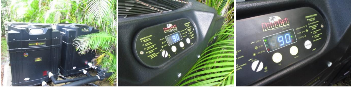
The Pool Heaters were functional
