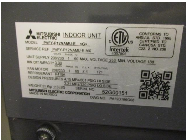
Air Handler Unit 5B (AHU 5B): Mitsubishi | 1 Ton | 2011 (installed in 2015) | The Air Handler is in the first-floor HVAC Room
