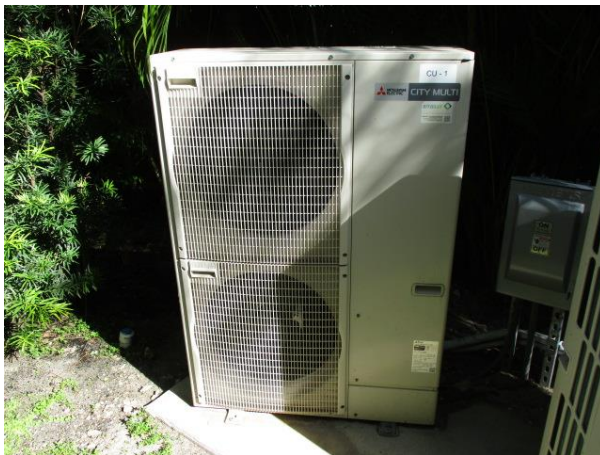
The 3 Ton Mitsubishi Condenser Unit 1 (CU 1) is at the North exterior Wall. It was manufactured in 2014 and was installed in 2015. It is paired with the two Air Handlers below.
