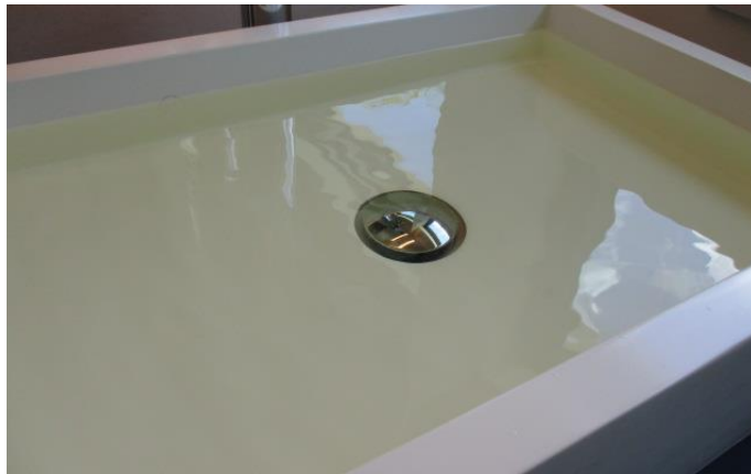
Slow draining was observed at the middle Upstairs Bathroom Sink.
