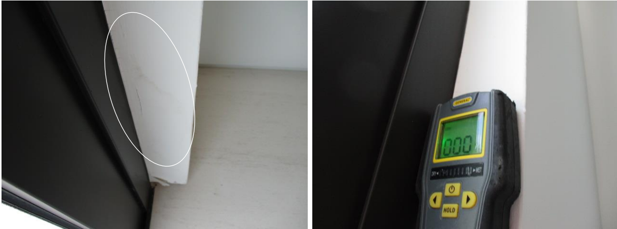
Water staining was observed at the bottom of the inactive sliding door wall frame at the middle Bedroom. This area was dry at inspection time. I recommend repair and remediation if necessary.
