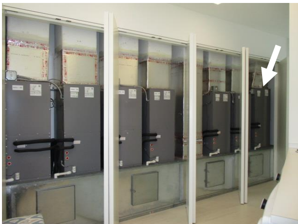
Air Handler Unit 5C (AHU 5C): Mitsubishi | 2.5 Ton | 2011 (installed in 2015) | The Air Handler is in the second-floor Utility Room
