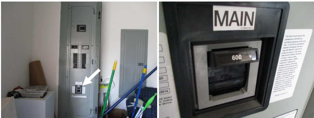
The 600 Amp Siemens Main Service Disconnect Panel is at the Garage West wall
