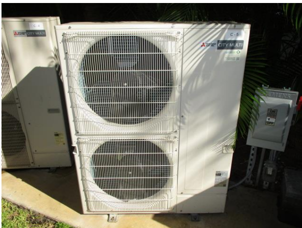
The 5 Ton Mitsubishi Condenser Unit 5 (C 5) is at the North exterior Wall. It was manufactured in 2014 and was installed in 2015. It is paired with the three Air Handlers below.
