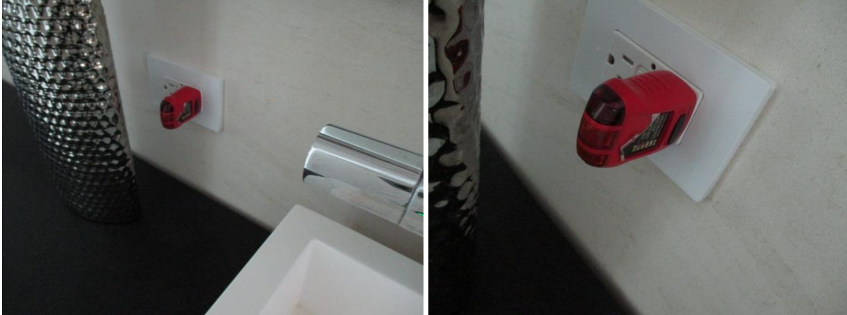
The GFCI Outlet next to the left Sink at the Master Bathroom is not functional.
