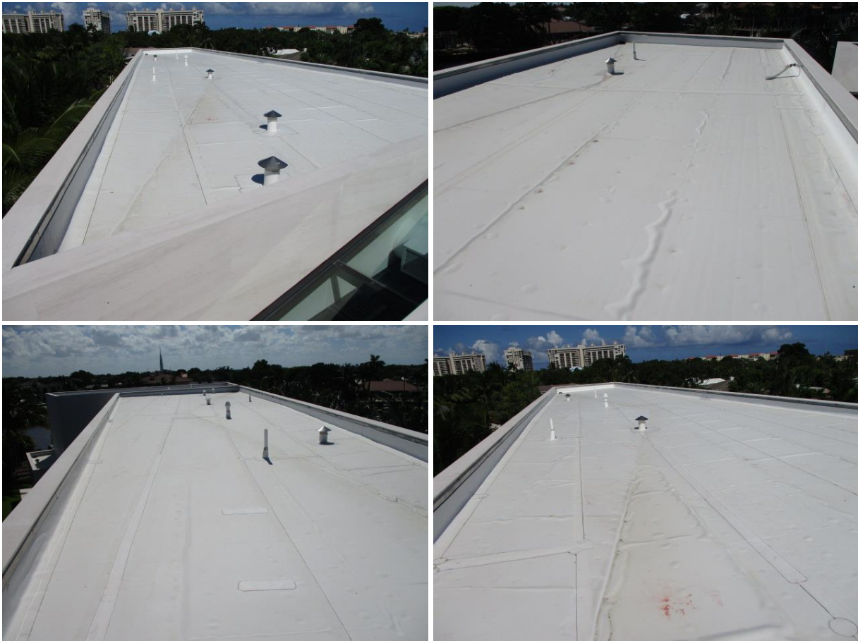
Roof style: Flat | Type of roof covering: PVC or TPO Single-Ply Membrane – good condition
