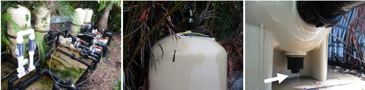
Leaking was observed at the Pool Filter, second from left, coming from the Gauge area. I recommend further evaluation and repair by a qualified pool technician.
