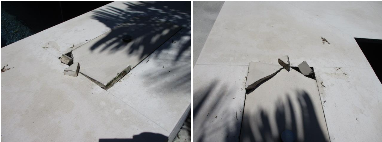
The decorative Limestone over a Cover Plate below the pool is cracked
