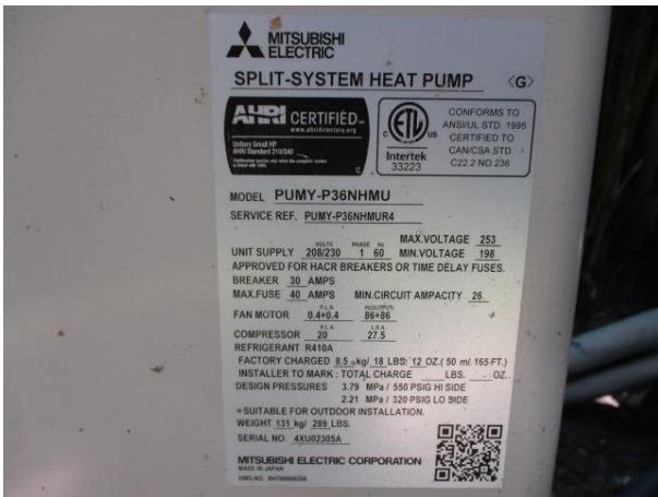
The 3 Ton Mitsubishi Condenser Unit 1 (CU 1) is at the North exterior Wall. It was manufactured in 2014 and was installed in 2015. It is paired with the two Air Handlers below.
