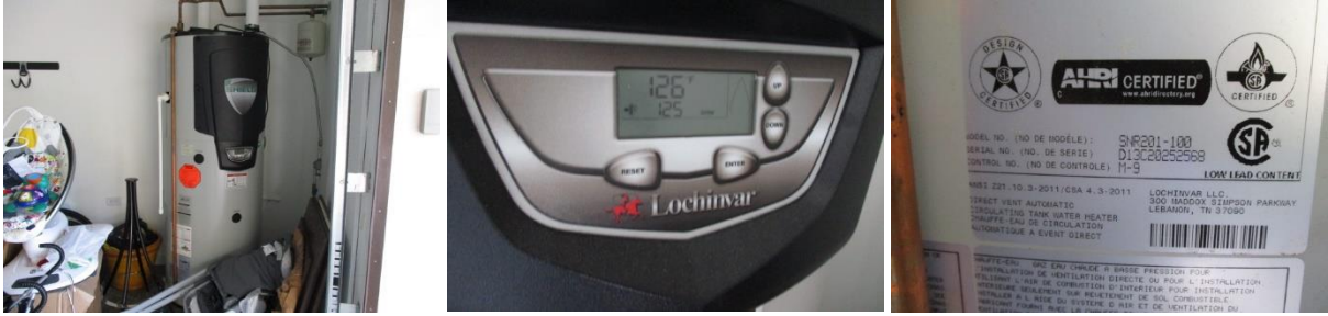
Water Heater: Lochinvar Shield (Commercial Grade) | 100 Gallon | Propane Gas | 2013 (installed in 2015)
