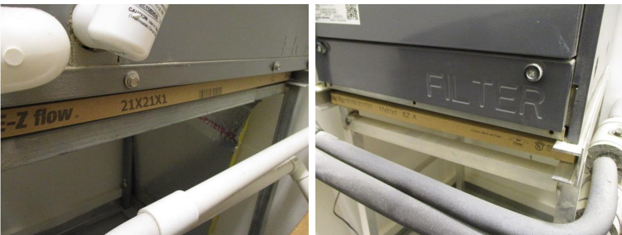
Filter Replacement Locations: At the bottom of Air Handlers
