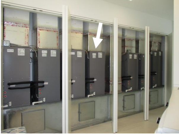
Air Handler Unit 4A (AHU 4A): Mitsubishi | 1.5 Ton | 2011 (installed in 2015) | The Air Handler is in the second-floor Utility Room
