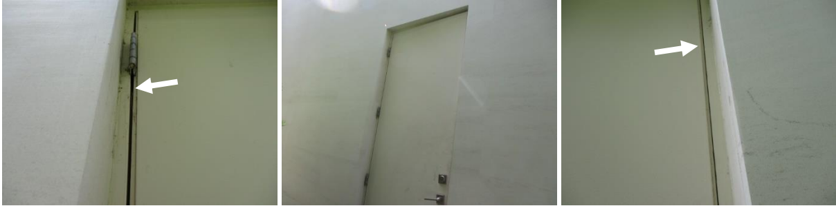
The North Side Exterior Door is tight at the frame. I recommend adjustment for better functioning.
