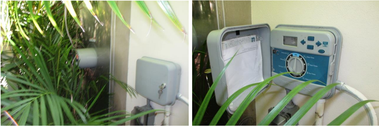
The Controller Panel is at the NE Property wall (left)
