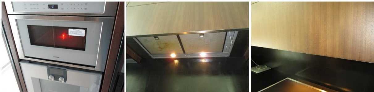
The Microwave Oven was checked with a Microwave Testing Device that illuminates when Microwaves are present in the Microwave Oven | The Hood Vent Fan and Light were functional
