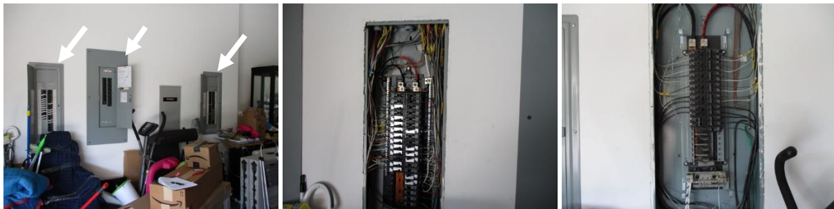
The three Siemens Sub-panels are in the Garage
