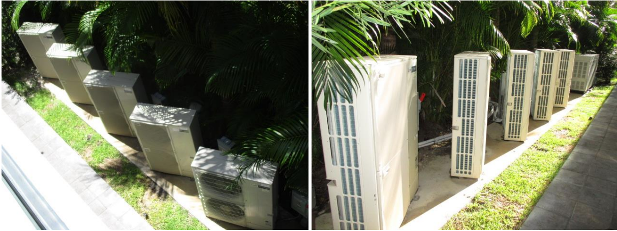
The Condensing Units (CU) are located at the North exterior wall. They are High-performance – High efficiency – low noise level Mitsubishi Citi Multi Series Condensers
