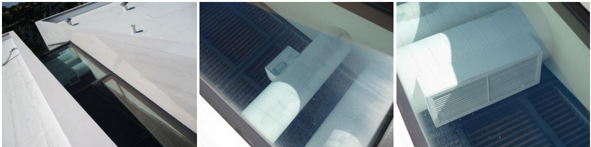
Visible components of the Duct System were observed from the Roof. Most Ducts were boxed-in or concealed above the ceilings
