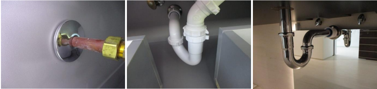
Fixture supply line material: Copper (left) | Fixture drain line material: PVC (center) & Stainless Steel (right)
