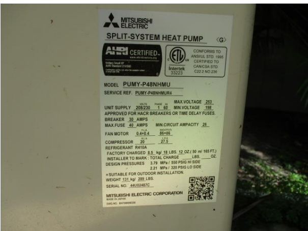
The 4 Ton Mitsubishi Condenser Unit 4 (C 4) is at the North exterior Wall. It was manufactured in 2014 and was installed in 2015. It is paired with the two Air Handlers below.
