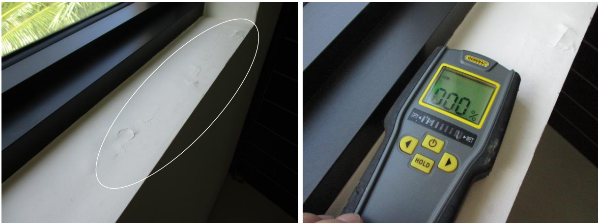
Water staining with some paint peeling was observed at the Window Sill at the "Jack & Jill" East Bathroom. This area was dry at inspection time. I recommend repair and remediation if necessary.
