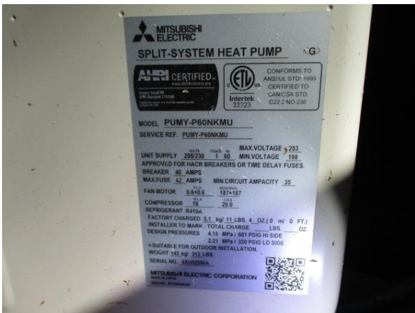
The 5 Ton Mitsubishi Condenser Unit 5 (C 5) is at the North exterior Wall. It was manufactured in 2014 and was installed in 2015. It is paired with the three Air Handlers below.
