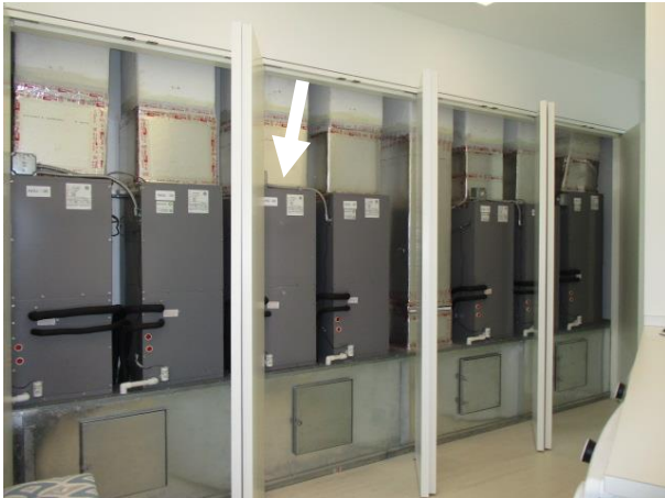
Air Handler Unit 4B (AHU 4B): Mitsubishi | 1 Ton | 2011 (installed in 2015) | The Air Handler is in the second-floor Utility Room
