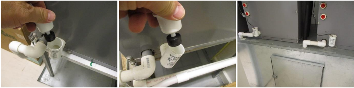
Condensation Float Switches (center) – these devices will shut down the Air Handlers when the condensation lines clog up. De-clogging the lines will allow the units to re-start
