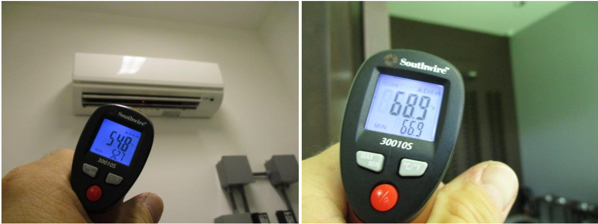
Two Mini Split Ductless Air Conditioners are installed in the Audio-Visual Room and the Pet Room
