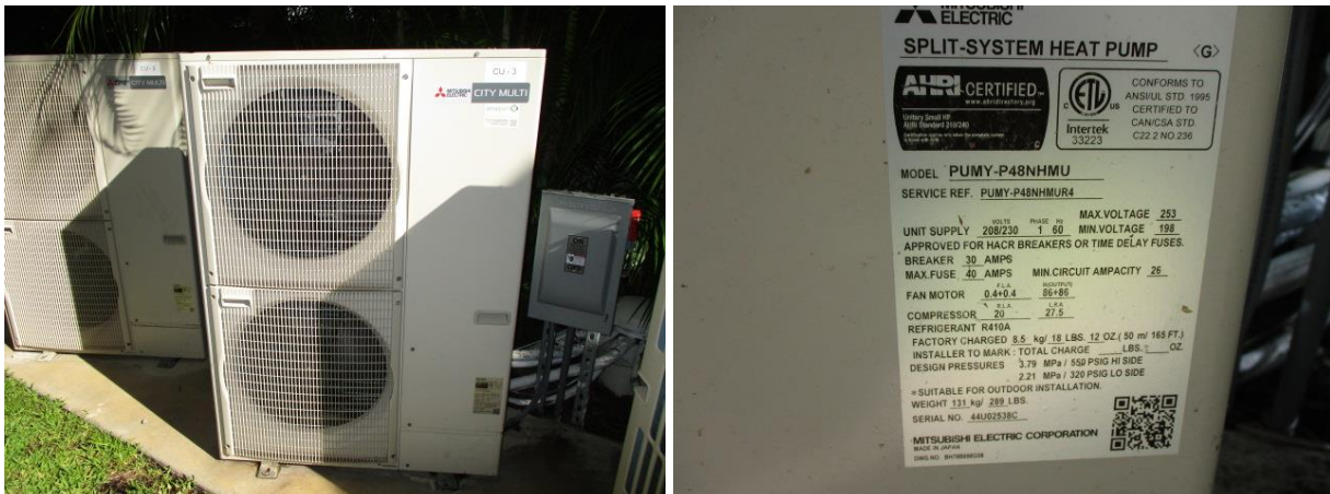
The 4 Ton Mitsubishi Condenser Unit 3 (CU 3) is at the North exterior Wall. It was manufactured in 2014 and was installed in 2015. It is paired with the two Air Handlers below.
