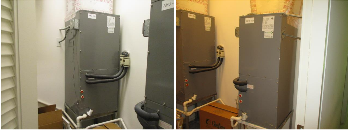
The Mitsubishi Air Handler Units (AHU) are in the second-floor Utility Room (seven) – top; at the first-floor Gym (one, under the stairwell) – middle; and in the first-floor HVAC Room, near the Garage (three) - bottom
