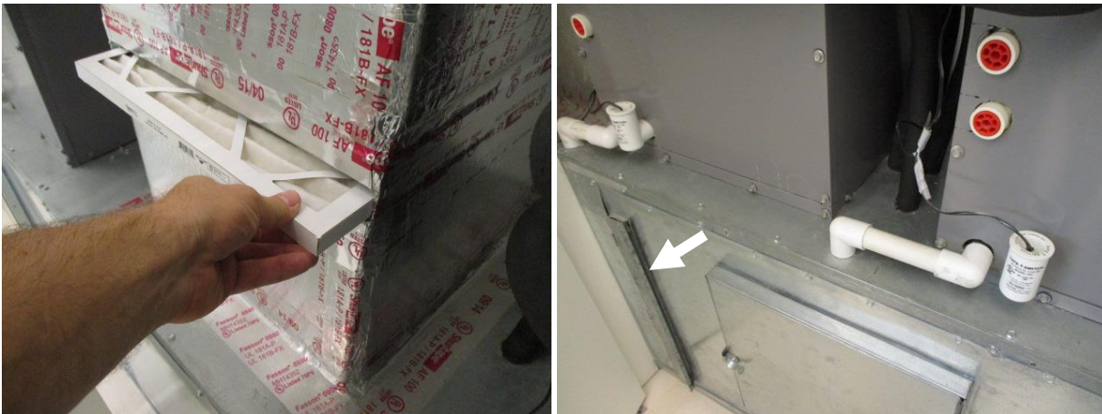
Filter Replacement Locations: At the Plenum, in the Utility Room
